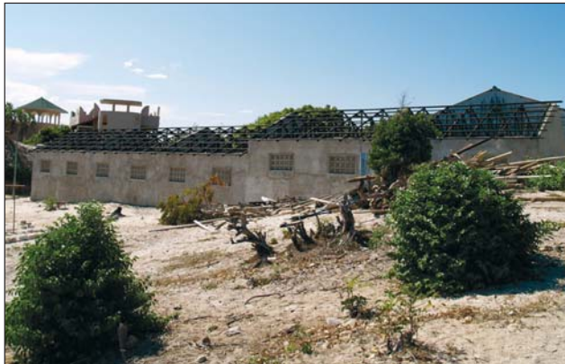
Roofless secondary school on 12/03/07. Note medicine bushes preserved in playground.
