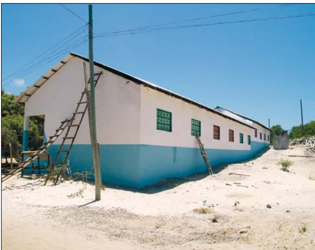
Finished secondary school on 22/03/07
