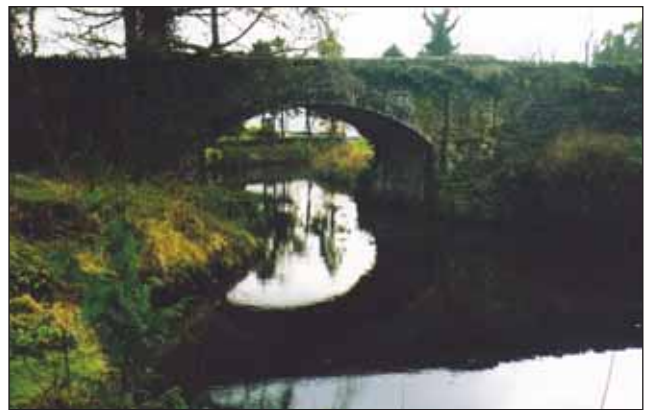
Canal bridge near Ballinamore
