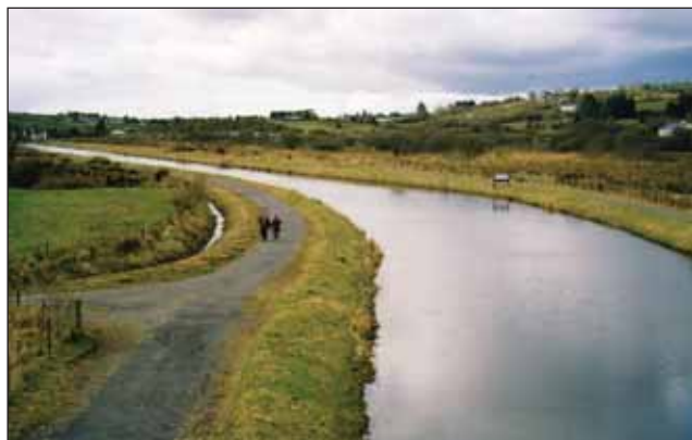
Walkway adjacent to the Boyle Canal
